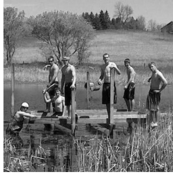
Repairing the wood dock on senior skip day in 2013
